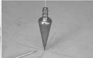
1. Drop a plumb bob from the center of the soffit to determine the column's center point on the floor. Mark this point for reference to align the column in the proper position under the soffit.
