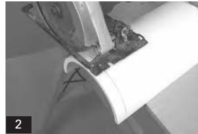
2. Always trim fiberglass columns from the bottom of the shaft using an abrasive cut-off blade. Make final adjustments with a belt sander or rasp.
