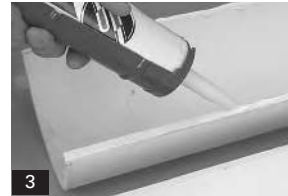
3. Insure the adjoining surfaces are clean and dry. Apply a bead of polyurethane adhesive to all connecting surfaces on both halves.
