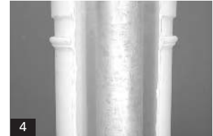
4. Align the column halves together around the structural support and join together.
