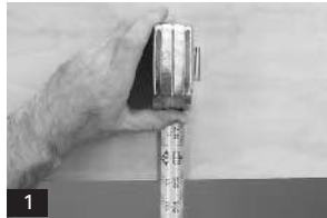
1. Measure the overall opening height.
