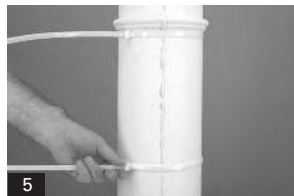
5. Secure using the straps provided in the Split Column Kit. Place straps approximately 18" apart and pull tight.
