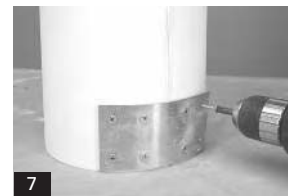
7. Install the joining plates at the top and bottom of each seam. Pre-drill pilot holes through the column and install the rust resistant screws provided in the Split Column Kit. NOTE: Plates are not required for wood columns.
