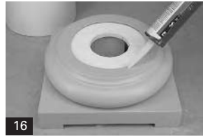
16. Apply a bead of paintable silicone sealant around the top perimeter of the base molding. Erect the shaft with the attached capital assembly onto the base.
