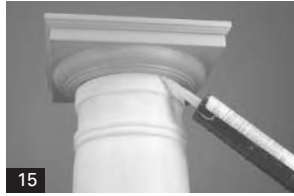
15. Apply a bead of paintable silicone sealant to the joint between the fiberglass capital and the shaft.
